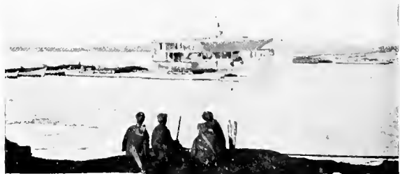
THE BRIDGE AT ARAB VILLAGE.
